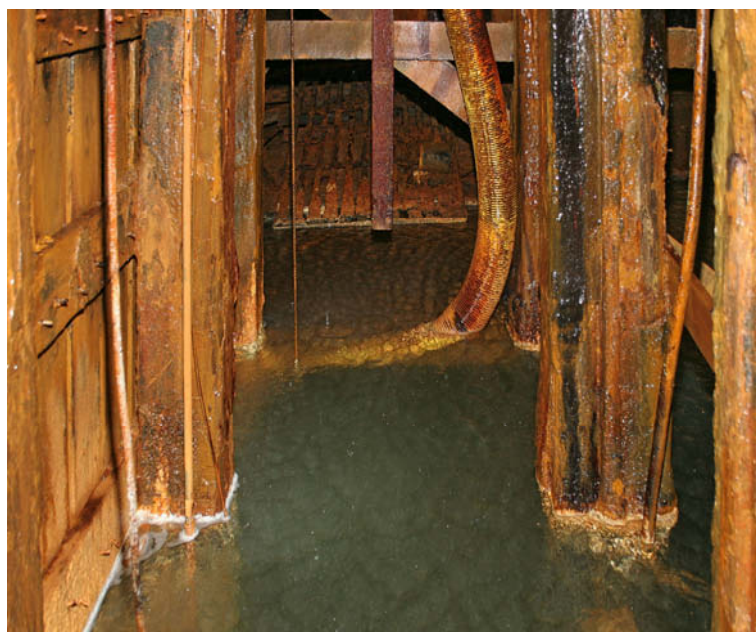
Fig. 15: The flooded Reiche Zeche shaft of the Freiberg/Saxony mining field (March 2 nd 2006). The brown colour is a result of ochre precipitates as a consequence of the catastrophic flooding of August 2002. Width of picture approximately 2 m.
