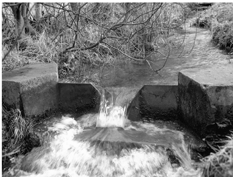
Fig. 49: V-notch weir measuring the flow of the Blaydon Hazard Shaft site near Newcastle upon Tyne, United Kingdom.
