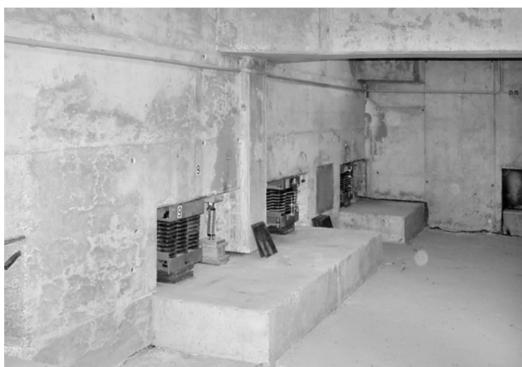
Fig. 34: Technical solution to secure a private house from destruction resulting from surface subsidence (courtesy Alexander Kattner, March 25 th 2003).
