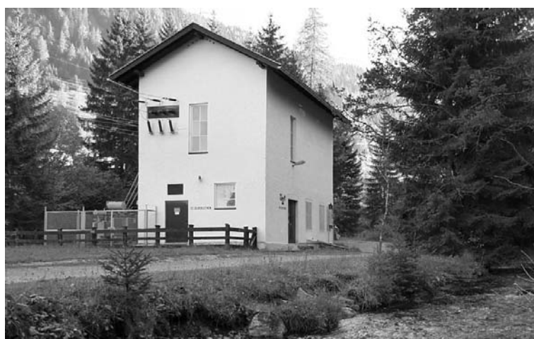
Fig. 12: Turbine house of the Austrian Biberwier/Tirol hydropower plant using mine water of the Max-Braun-Adit located in the Silberleithe hills that can be seen in the background of the photograph. The first turbine to produce energy was installed in 1904; the currently operating turbine was installed in 1936.
