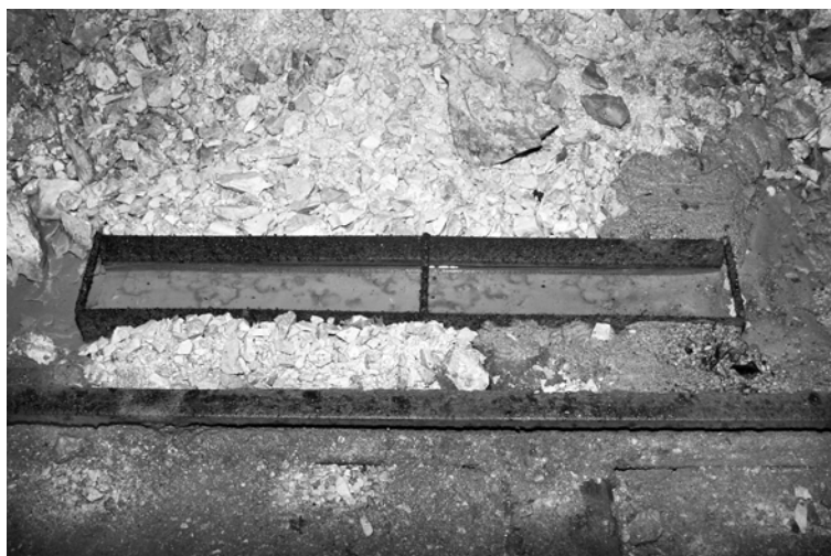
Fig. 50: Badly maintained channel for flow measurements. The channel inflow is not laminar and the channel itself is filled with sediment.
