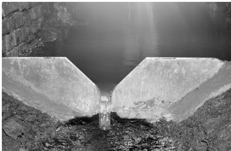
Fig. 55: A V-notch weir in the Felsendome Rabenstein/Germany underground visitor mine showing that the sharp crested side has to be at the upstream side of the weir.
