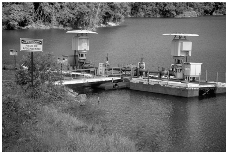
Fig. 32: Settlement lagoon and drainage pumps of an open pit iron mine near Belo Horizonte/Brazil.
